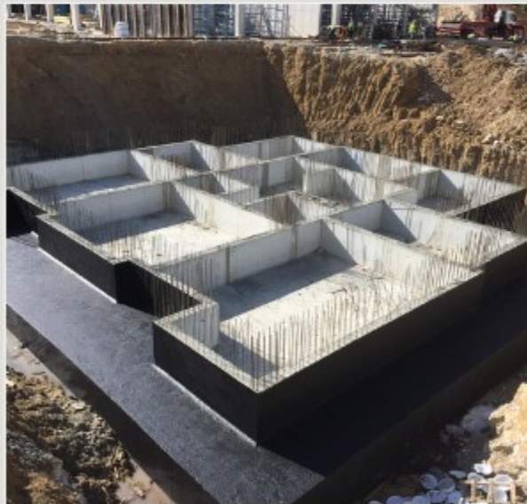
Foundation Hydro Isolation
