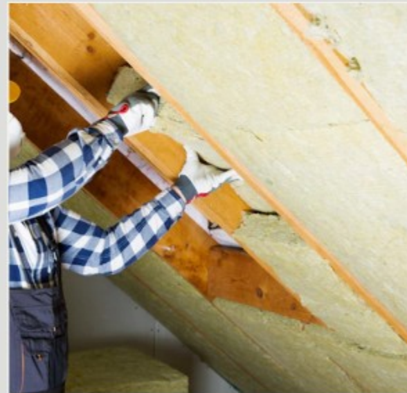
Roof Thermal Insulation
